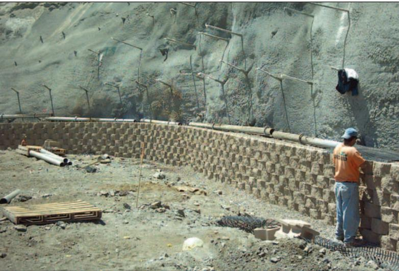
After those nails were placed, the sacrificial nail had to be sealed. Each boring was pressure grouted until all of the air was removed. This process ensured that the galvanized nail did not erode due to moisture contact. The slope face was then shotcreted to prevent erosion or slope failure. Next, the top half of the ramp was removed in order to access the middle portion of the slope and the soil nailing and shotcreting process was repeated.
