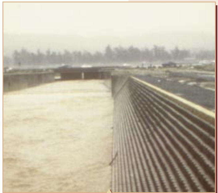
Phase I of Peter's Canyon Wash is complete.
