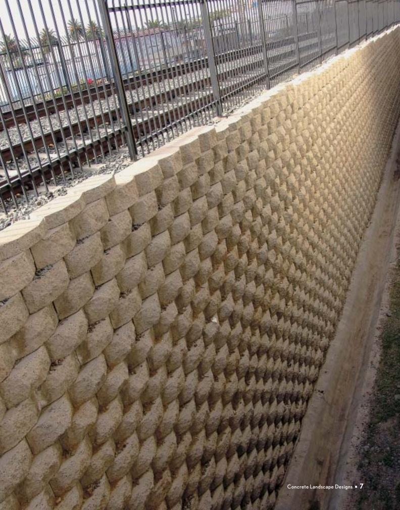
greater with six inches (152 mm) of well-compacted granular fill. Because the bottom of the wall was sitting on poor soil matter, the whole base was reinforced with geogrid.
