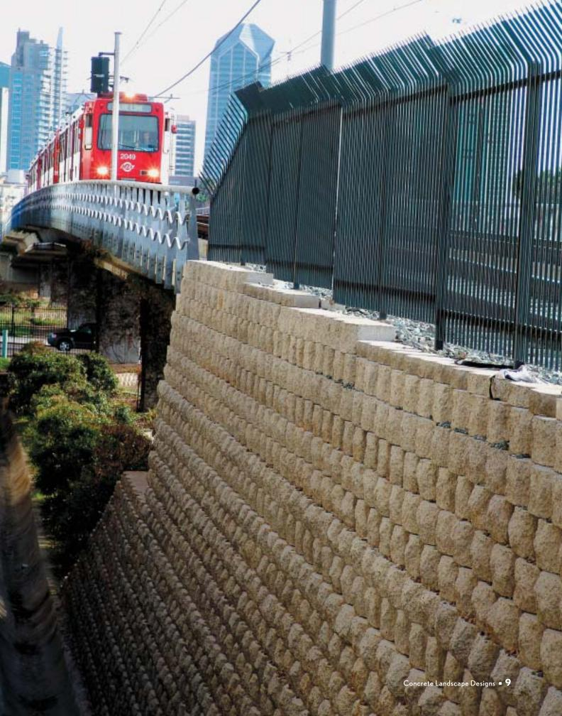
Haggerty also said that besides costs savings, MTDB made the choice to use a segmental retaining wall system because it allowed them to use a more vertical pattern than the original system that had been specified. The site called for a near-vertical wall to fit into the space and segmental retaining walls were able to solve this building challenge.
